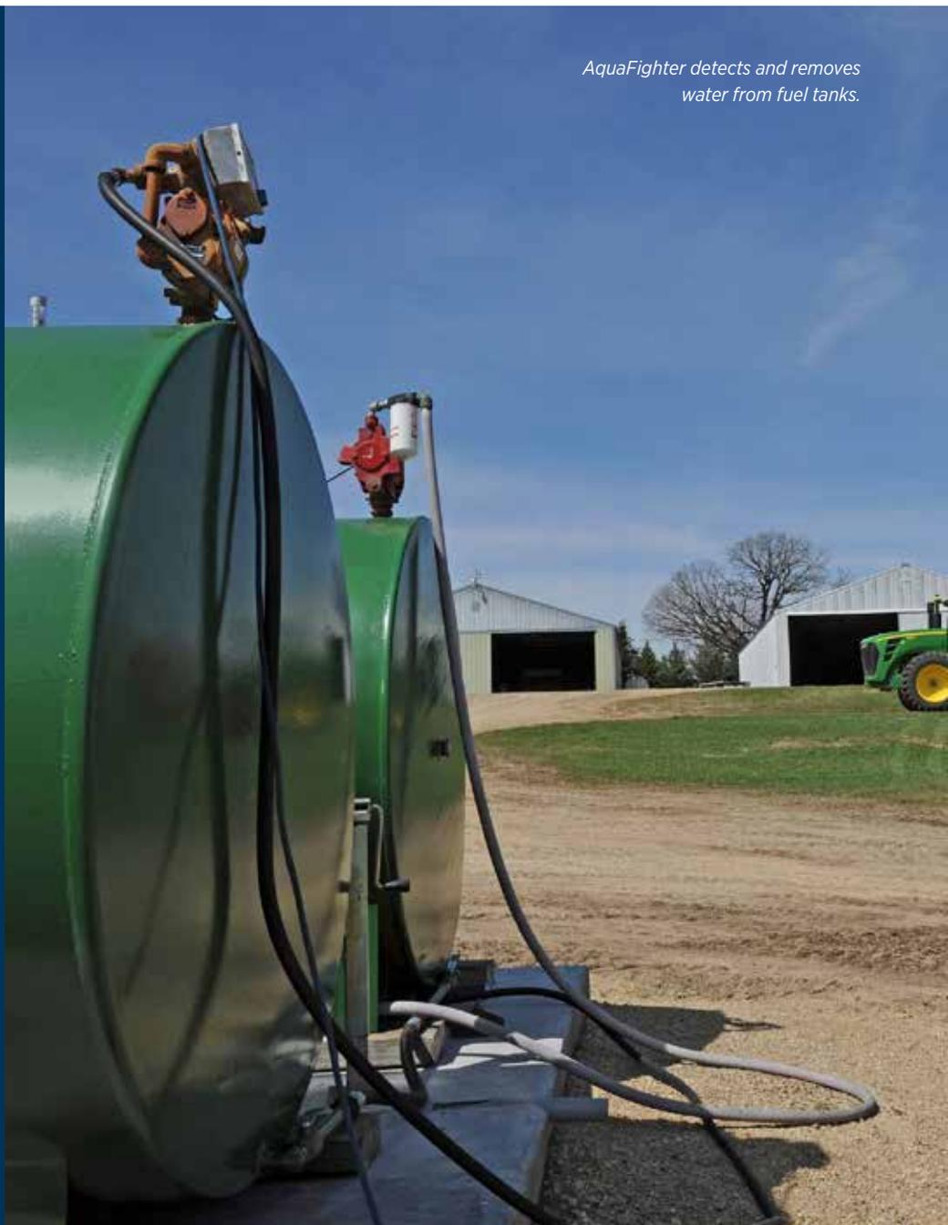
*AquaFighter detects and removes water from fuel tanks.*
